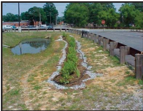
Completed rain garden at DSCR for stormwater control.
